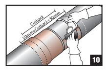
Using a brush or roller apply the coating to the joint area to the required thickness, covering at least 50mm of the mainline coating, on each side of the joint area. Ideally, coating should be only applied at temperatures above 15°C and 3°c above dewpoint. For low temperature applications consult a SPC engineer.
