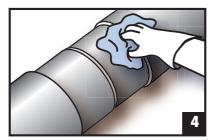
Clean exposed steel and adjacent pipe coating with a non oily cleanser - eg: MEK - to remove the presence of oil, grease and other contaminants Do not use paint thinners.
